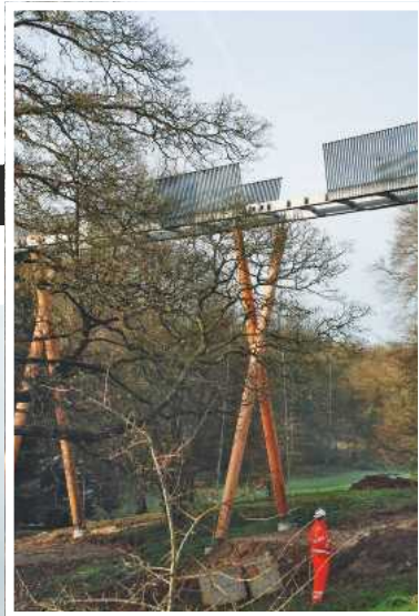
A glimpse of the new walkway, which is coming along nicely
